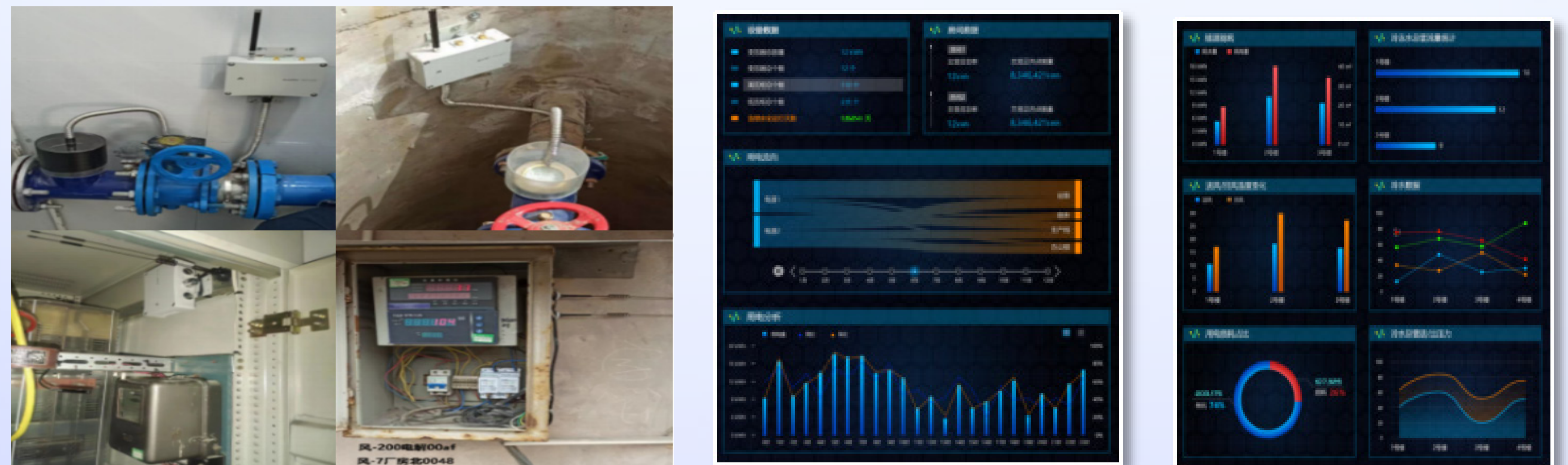
5G-Based Energy Consumption Data Collection and Back-End Data Monitoring and Analysis
